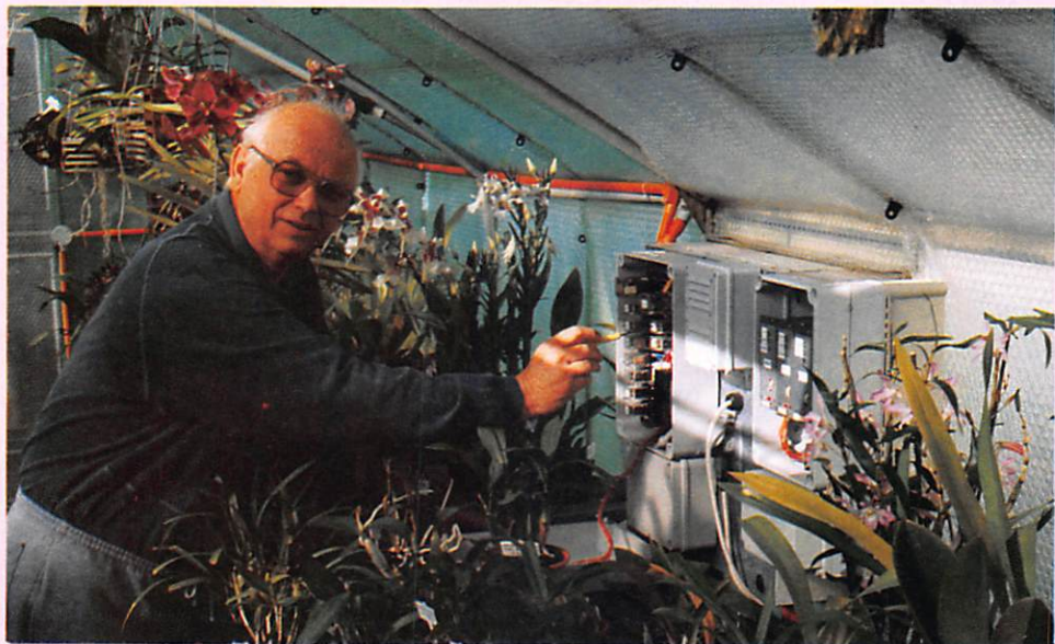
Bernie Killington adjusting electronic controls in glasshouse
